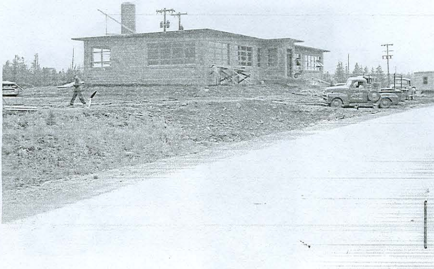
Construction was started on 13 September 1955 View taken on 11 July 1956
